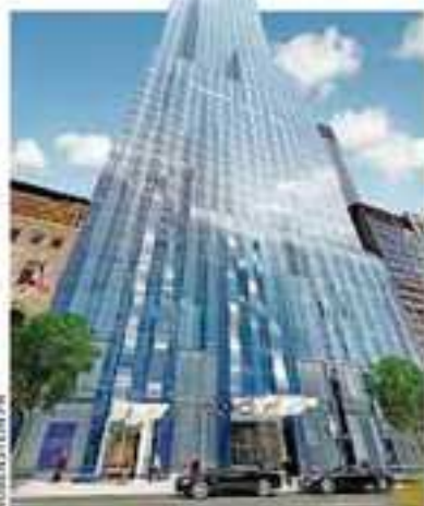
One57 from Extell is a pre-construction hit
